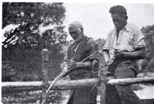
Te Kehu (left) and Tau Tamakehu lash the top rail of the fence with split kareao.
