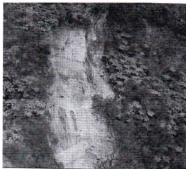
The Mangapurua slip, about 60m wide, tore a massive hole in the bush. It was in an area which had not previously been known for slipping.
